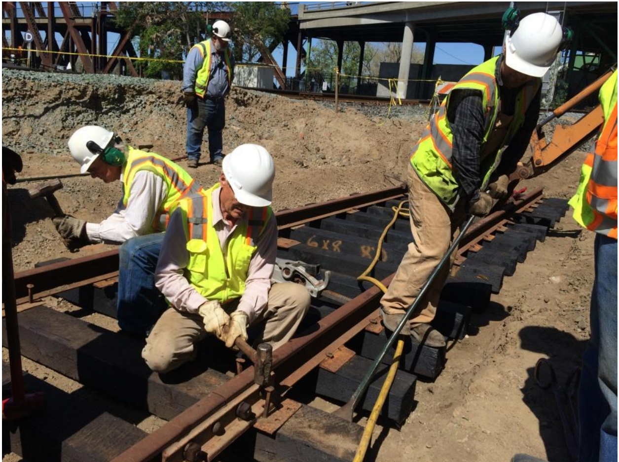
Steve and Kent set the spikes at the joints, which had to be driven by hand, while DJ nips the tie
