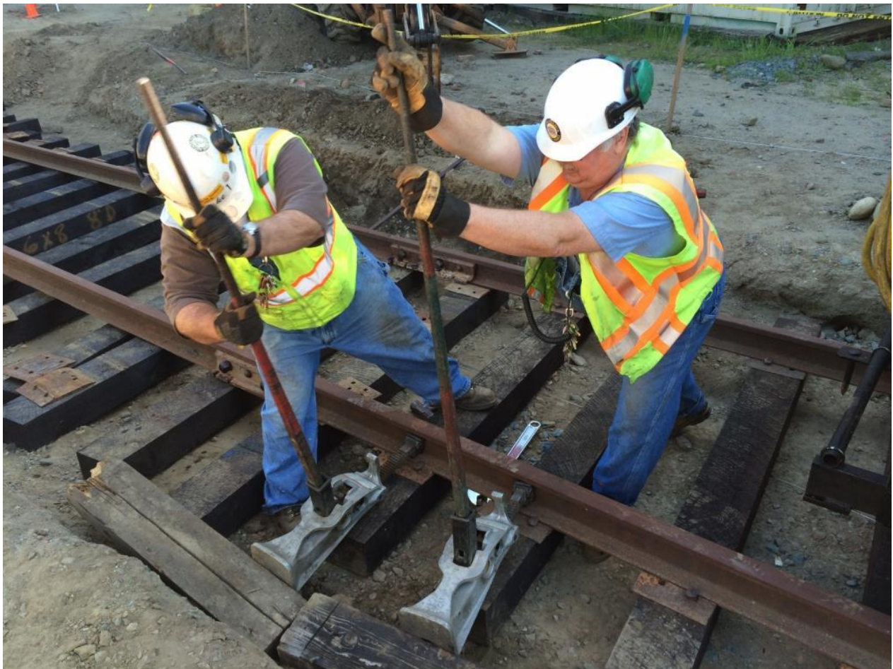
Now Mike F. and Chris put the curve in the track
