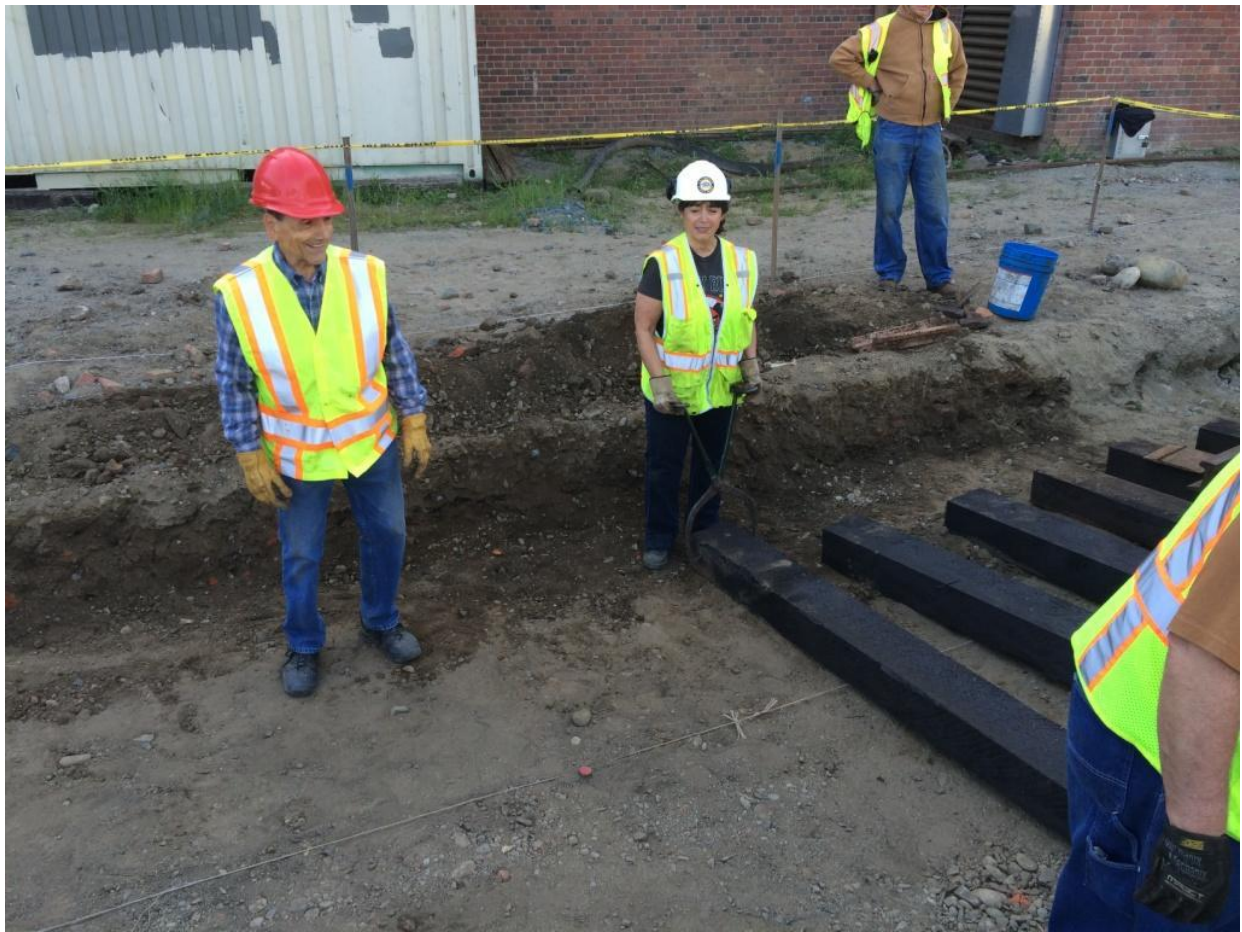
Harry G. and Pam set out the ties for the final panel of track
