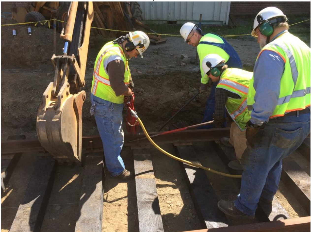
Mike F., Dave, DJ, and Frank start spiking the east rail off of which we'll gauge the track
