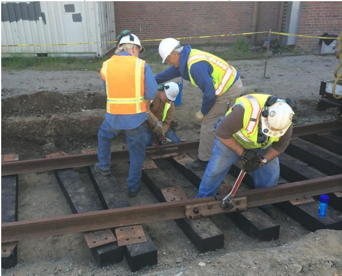
With the final two rails in place, Fred, Steve, Kent, and Mike F. bolt the joints
