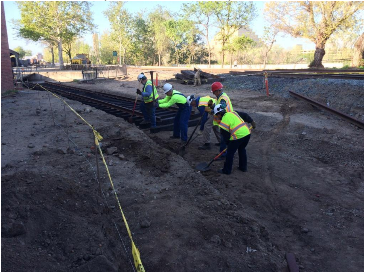
“Drill, Ye Tarriers, Drill” Frank, Dave, Kent, Harry G. and Pam make the final cut in the bank for the proper curve
